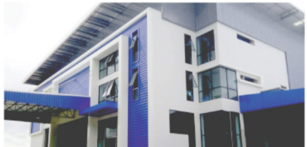
Refrigeration System Manufacturing Plant
